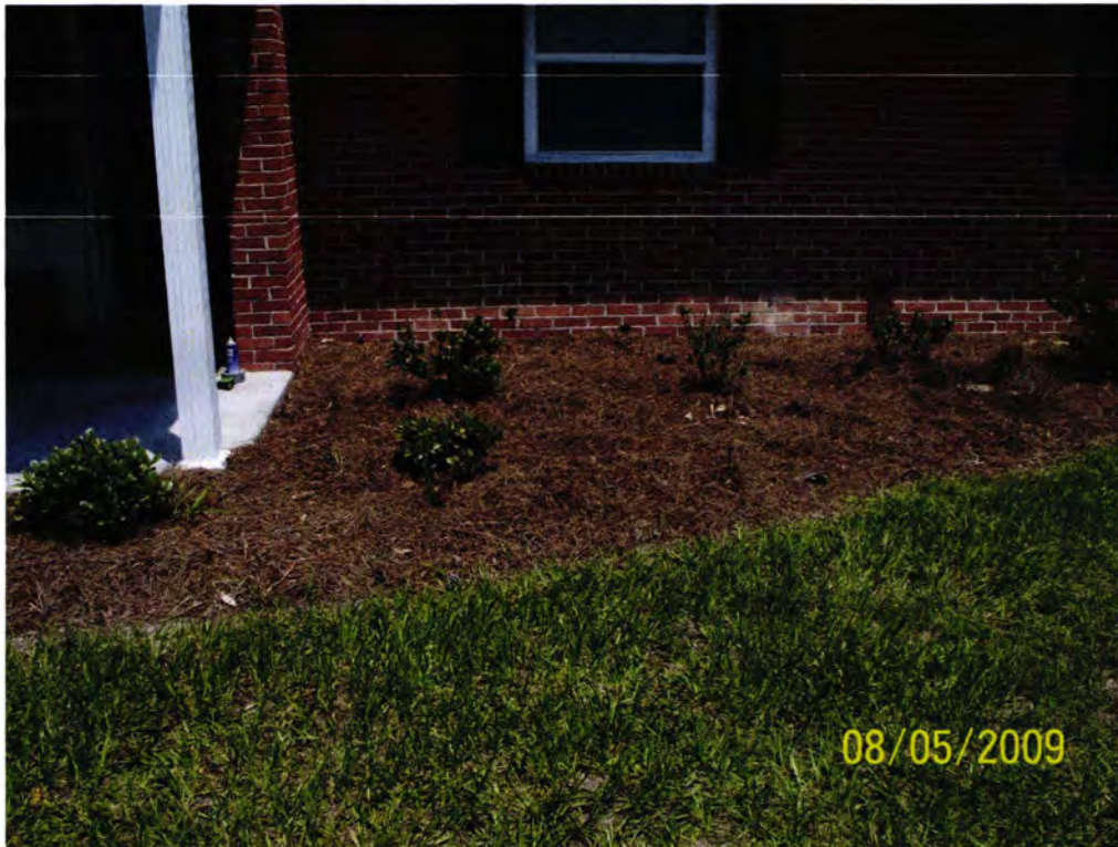
Picture 1: Location of UST 1434Dove.
