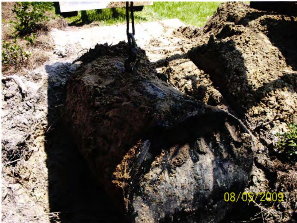
Picture 2: UST 1434Dove.
